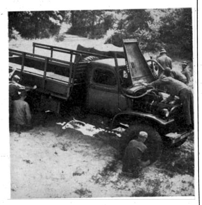
A VERITABLE BEEHIVE OF ACTIVITY precedes the actual streamcrossing. Automotive students, briefed by a department instructor, make a close inspection of the waterproofed two-and-a-half-ton truck to be sure all points are sealed. The truck forded the stream smoothly and in record time.
