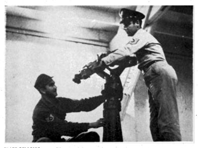
**EMERGENCIES** . . . They can be a trying job, particularly when accidents are infrequent. Here two Crash Crew members inspect the cut-off valve of a turret nozzle on a 155 Aircraft Crash Rescue Truck. (Dept. of Defense, U. S. AIR Force Photo).
