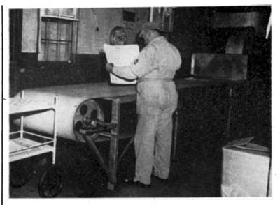
AFTER THE POSTERS come through the dryer, Sfc. Walter E. Spencer removes them from the conveyor belt and stacks them. After one run is completed, the screen will be cleaned, a new stencil put in place, and the cardboards go through this same process again.
