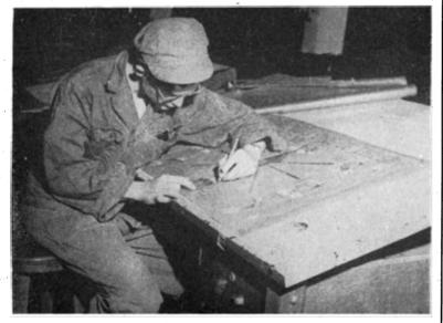
ONE OF THE MOST DELICATE TASKS in making a poster is cutting the stencil. The nearly transparent stencil is laid over the original painting, and the top layer of the stencil is cut away. For this particular poster, five stencils will have to be cut—one for each color to be used.
