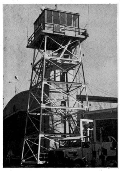
**LAWSON PULSE**—The control tower at Lawson Field, an integral part of Fort Benning, is the guiding hand of all aircraft landing and taking off from the Post. Operated by Airways and Air Communications personnel, the tower provides the latest weather data, field clearance, and landing and take-off obstacles to all military aircraft in the vicinity.
