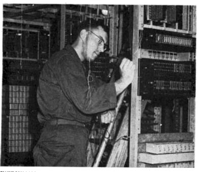
**SWITCHMAN PVT. D. R. SKENDER,** 3440th Area Service Unit, has the job of keeping the machinery for dial telephones in order.
